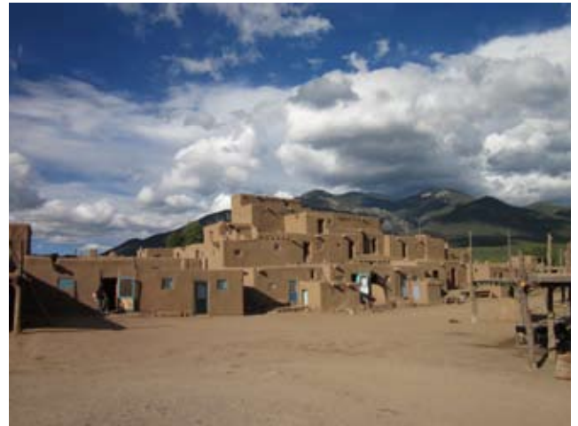
Taos Pueblo has resisted architectural change for the last century. Restrictions against utilities have resulted in usage of homes for traditional activities over daily life. The five-story buildings are still maintained with traditional mud plaster. Photo by Shawn Evans.
